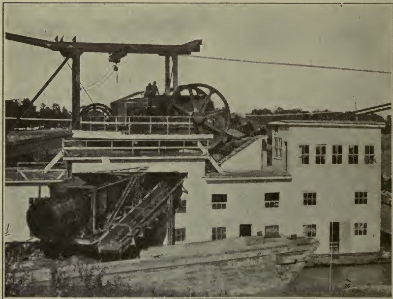
Fig. 56. Ladder Dredge Provided with Trough for Discharging Excavation into Barges
